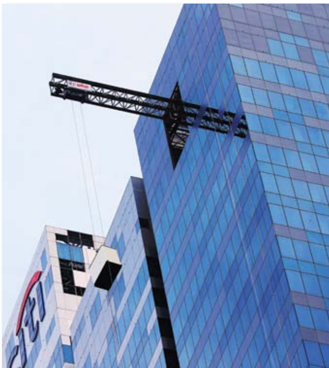
A winch trolley is moving out Asia's Square's façade on MHE-Demag's hoisting system, paying out a hook for some heavy lifting.
