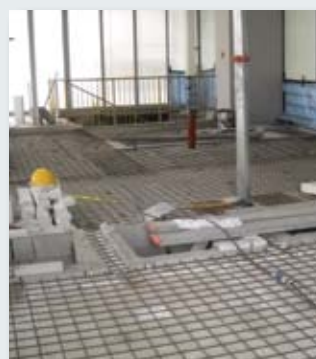
Construction site at a five-star kitchen: JEOFOAM is applied to raise the kitchen floor some 430mm. The light-weight foam forms the ideal fill material.
